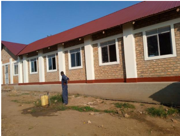
New Building after Completion
