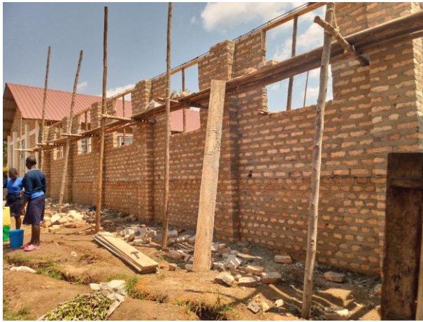
Building at Beam Level
