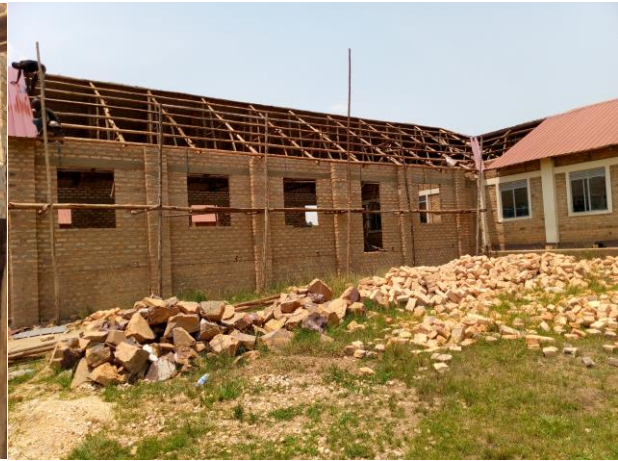
Building being Roofed
