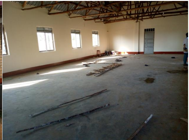
Inside the New Dormitory
