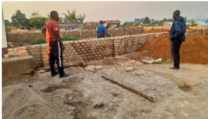
New Dormitory at Foundation
